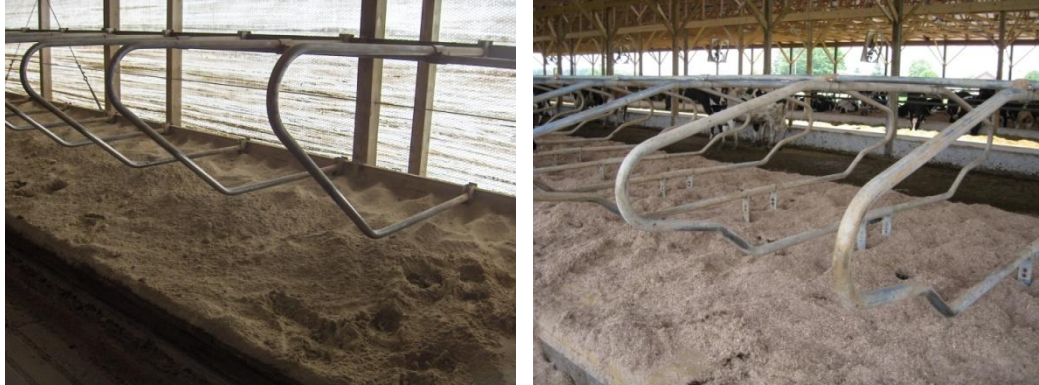
Figure 2. Deep bedding minimizes potential for hock injuries, improves stall usage, and increases lying times.
