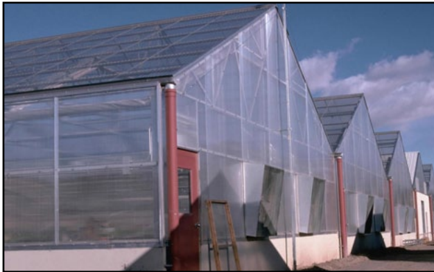
EXTERIOR OF GLASS-COVERED CONVENTIONAL GREENHOUSES.
