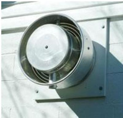
**Choose a well-ventilated room where temperatures are controlled.** Exhaust fans directed to the outside of the building reduce the buildup of noxious vapors from many of the solvents used in pesticide formulations. Ventilating the pesticide storage room into an adjoining room does little to solve the problem. Pesticide labeling often gives temperature limits for storing a product.
