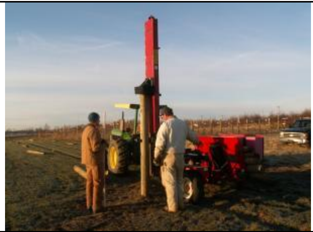
Figure 2. Driving in posts at marked locations
