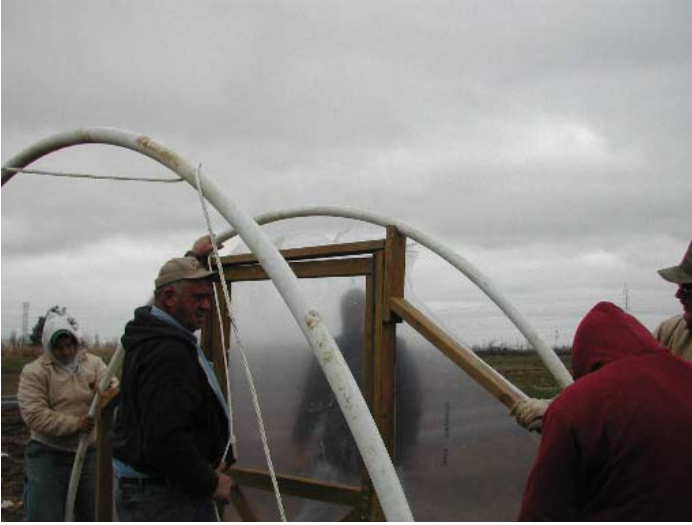
Figure 6. The Endwall is Placed Under the Last Hoop of the Tunnel.
