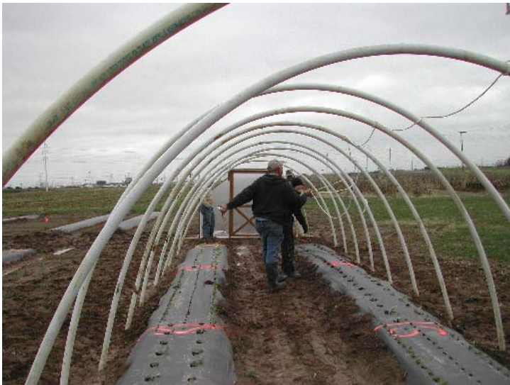
Figure 5. The Rope is Being Run Off Center Throughout the House For Added Stability.
