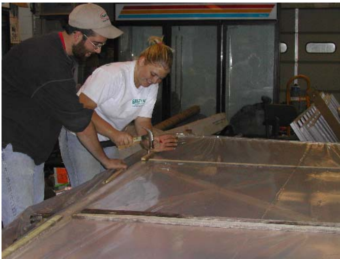
Figure 1. Attaching plastic to the endwalls using wood, hammer, and nails.
