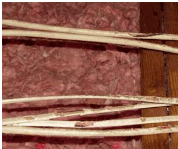
Wiring chewed by rats (photo: tristatewildlife.com)
