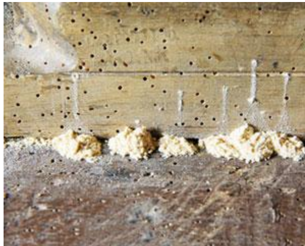
Powderpost beetle "shotholes" and sawdust (townandcountrysolutions.com)
