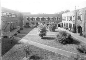
9. The Engineering Quad
