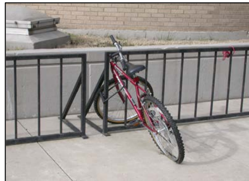
"Wheelbender" racks do not support the frame of the bicycle, potentially damaging the front wheel.
