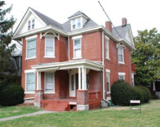
Existing Transylvania Park Character
