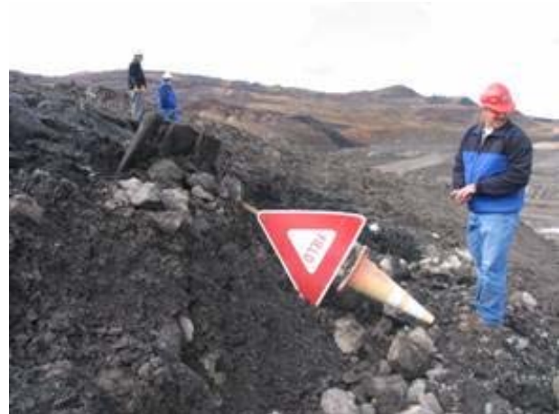
Figure 2. Upturned sign on a haul road uplifted by the landslide toe.
