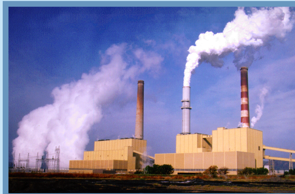
At power plants, limestone is used in "scrubbers" to reduce air pollution.
