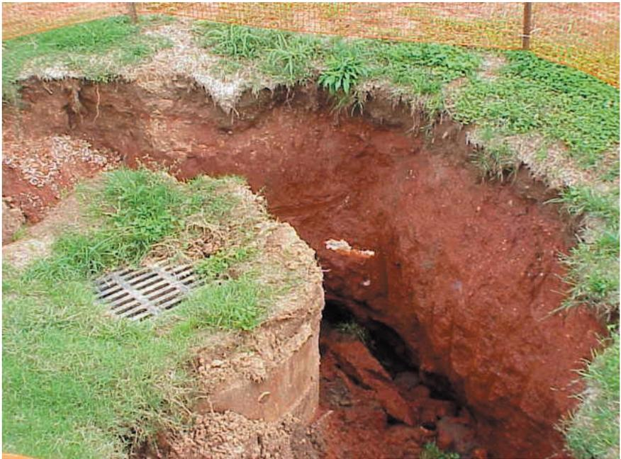
Figure 9. Surface collapse around dry well in Bowling Green, Ky. Hole is approximately 5 feet deep.
