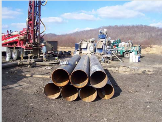
Surface Casing Rig
