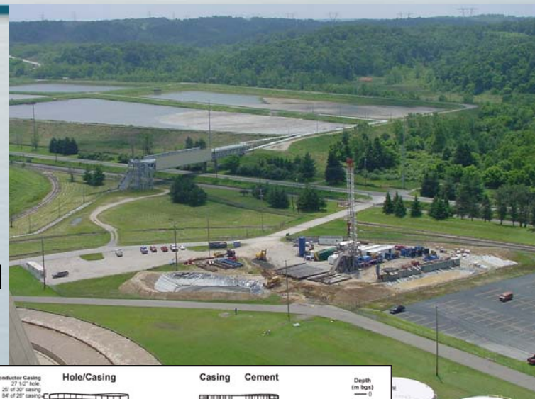
Drilling Test Well
