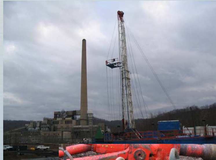
Deep Well Rig
