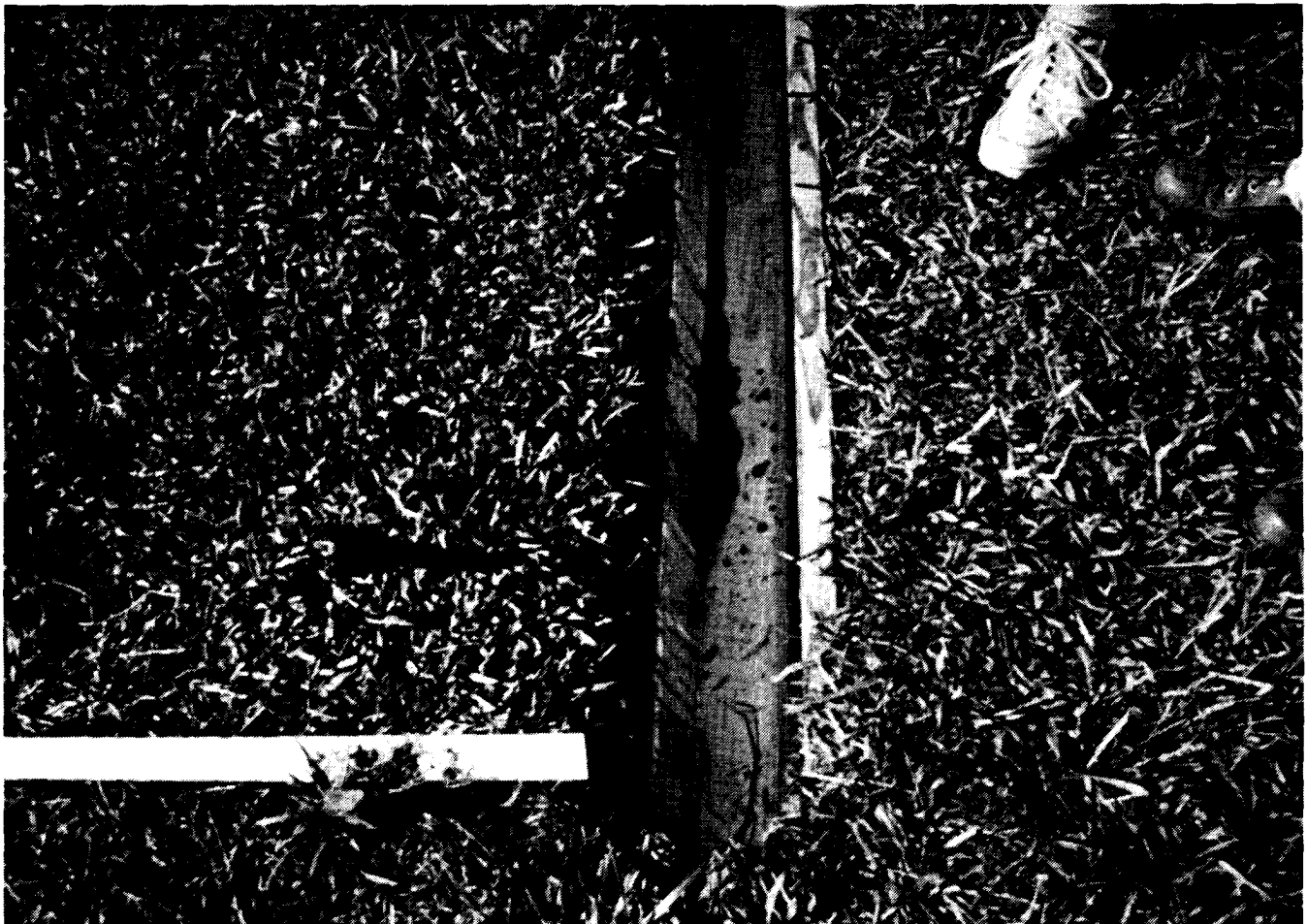
Figure 5. Gutter below filter strip.
