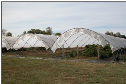
MULTI-BAY QUONSET (HAYGROVE) TUNNEL
