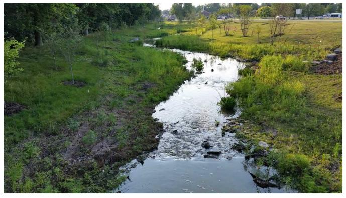
After filling and grading the floodplain, sowing seed, planting new trees, and waiting four months, Big Elm Fork looks more like a natural stream and can spread out over a wider floodplain during storms.
