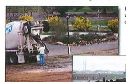
Figure 1. Chute washwater being dumped on the ground
