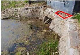
Lower Basin (3.1): The outfall inlet of the basin was cleared of obstructions to ensure proper flow.
