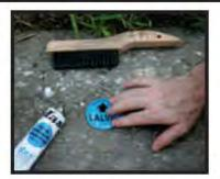
Place the marker on the application surface. Push down HARD with a twisting motion, forcing adhesive out from the edge. It is important that the entire edge of the marker is sealed to the application surface.
