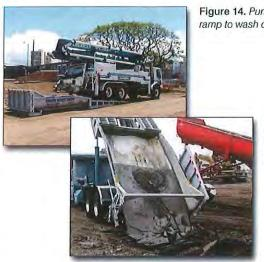
Figure 14. Pump truck using the ramp to wash out into a roll-off bin
