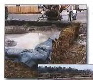
Figure 9. Hay bale and plastic washout pit
