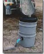
Figure 3. Concrete washout filter
