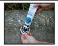
Apply adhesive to the back of the marker as shown. Start 1/8" in from the outside edge, applying an even bead around the entire edge, and then work to the center.
