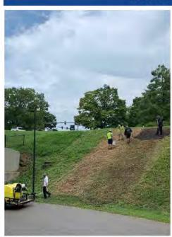
UK Grounds is transforming the slopes on either side of the Cooper Drive pedestrian underpass (left) to improve maintenance conditions by restoring the ecological function of the vegetation in this area. The turf grass is being replaced by native grasses and plants to create the University's largest pollinator habitat. The deeper rooted native plants and lack of mowing will also provide erosion control improving stormwater quality and reducing run-off. Grounds is
