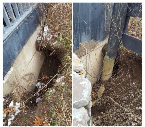
Upper Basin (3.5): There are two growing cavities around the basins outlet structure.
