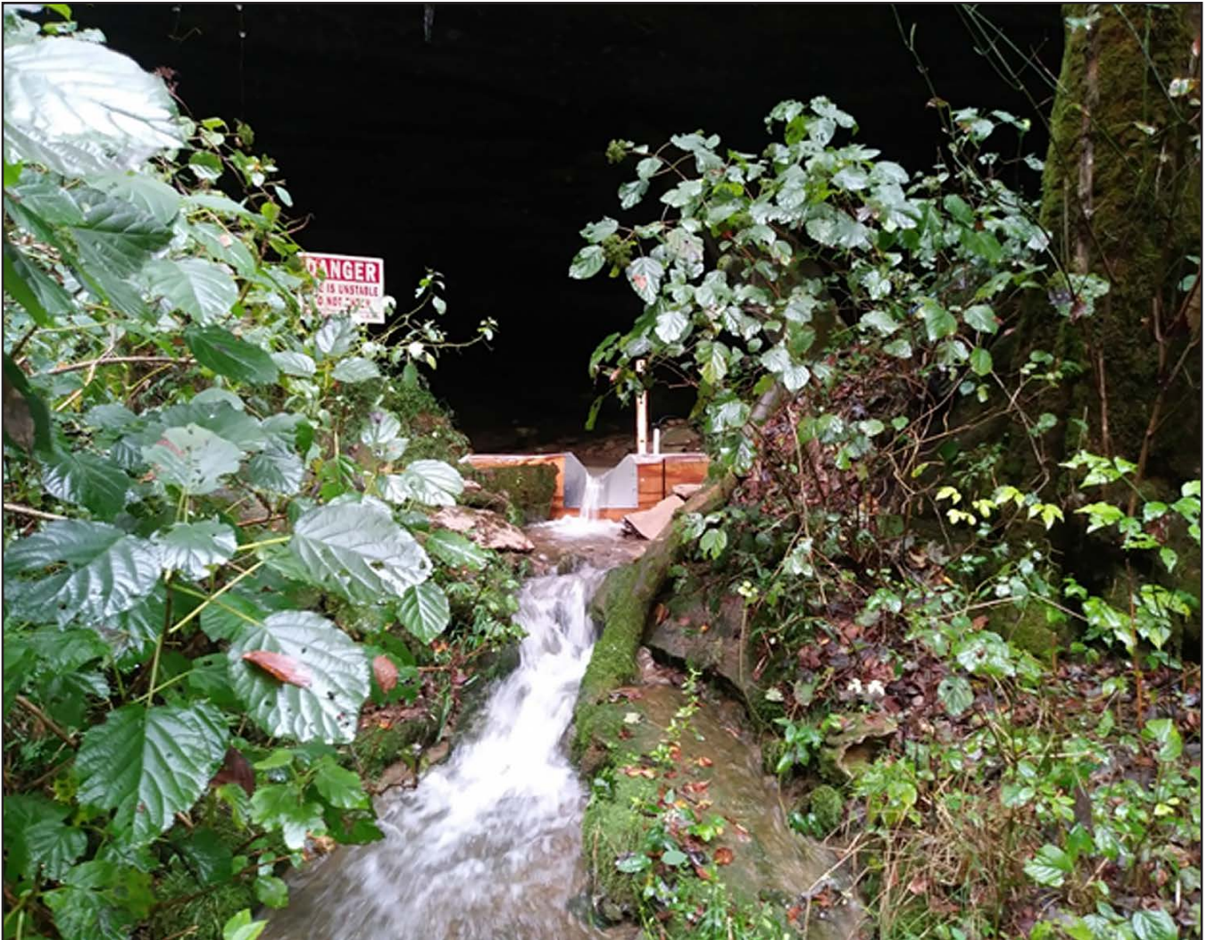
Figure 7. Weir installed to measure flow rate at a karst spring at The Homeplace on Green River as part of a project to characterize the karst hydrogeology of the area.
