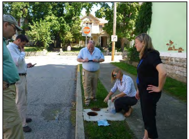
Figure 5. From left: Mike Unthank (U.S. Geological Survey), Craig Frye (Northern Kentucky Sanitation District), Scotty Robertson (Division of Water), Catherine Fargen (U.S. Geological Survey), and Brooke Shireman (Northern Kentucky Sanitation District) inspect the test well at the Bellevue site.
