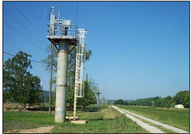
Figure 9. A public water-supply well near the Ohio River in west-central Kentucky.
