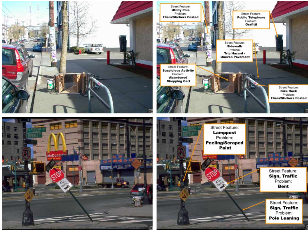
Figure 6. Residents would be asked to use their feature-conditions sheets to practice identifying things in the urban scene that need to be recorded in the handheld device. Source: Sustainable Seattle (2004).
