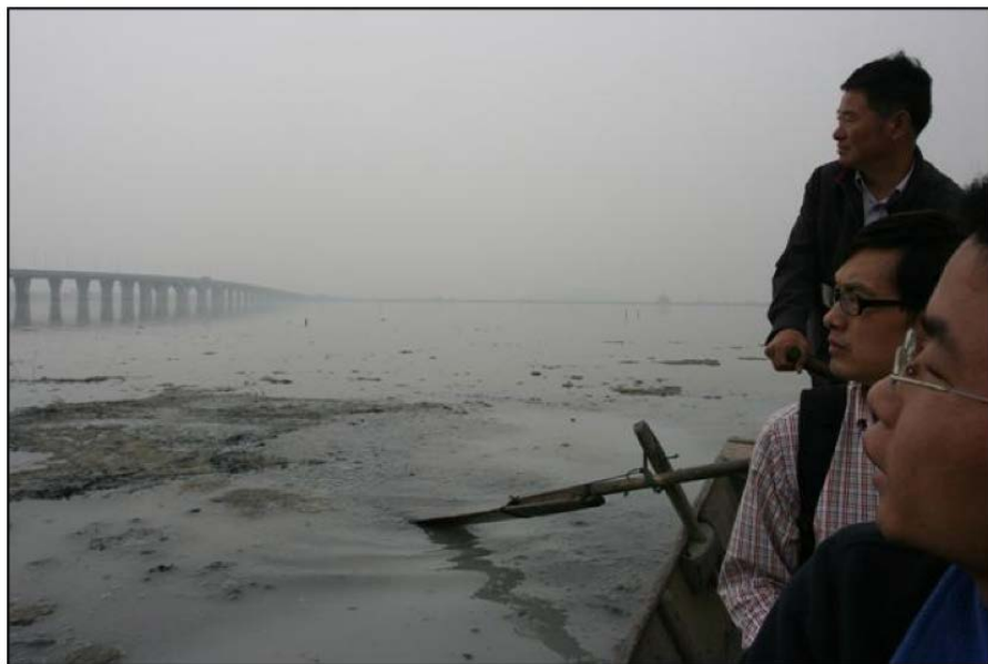
Figure 5: On-site Investigation, Photo: Ma Jun
