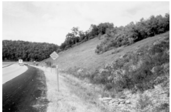
Figure 2. Highway Right-of-Way (Photo by A. D. Luscher).
