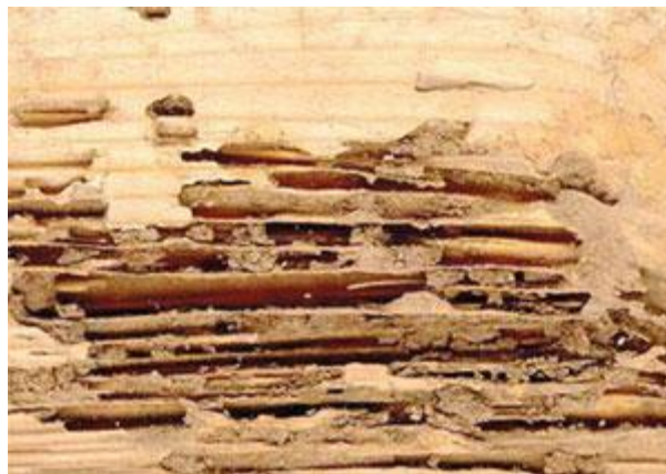
Soil in termite galleries in wood (www.narragansetpestcontrol.com)
