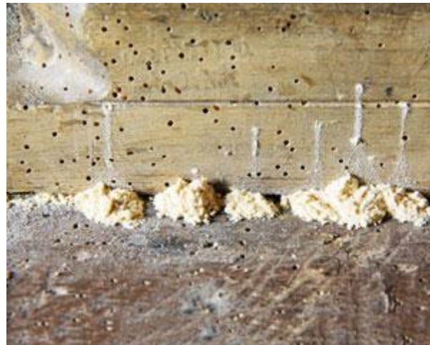
Powderpost beetle "shotholes" and sawdust (townandcountrysolutions.com)
