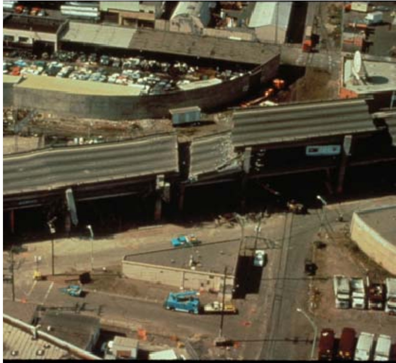
Figure 1-4. I-80 damage during the 1989 Loma Prieta earthquake
