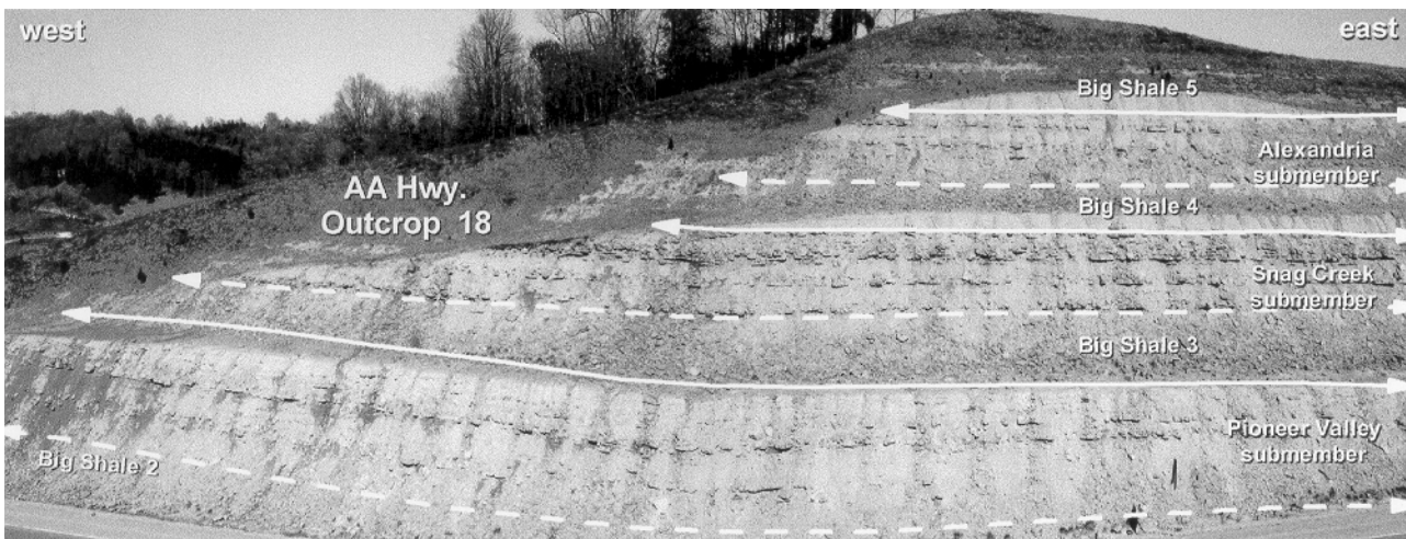
Figure 8. AA Highway Outcrop 18. Section through lower and middle Kope Formation (lower Pioneer Valley through lower Grand View submembers); note good development of decameter-scale cyclicity. The two benches in roadcut on north side of highway are at the level of “Big Shales” 3 and 4.
