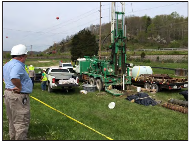
Figure 5. Scotty Robertson observes the installation of a monitoring well at the Big Sandy Power Plant, located along the Ohio River near Louisa.
