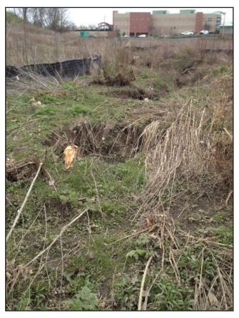
*Figure 6. In-stream sinkholes in the proposed stormwater detention basin site at Old Brownsboro Crossing.*
