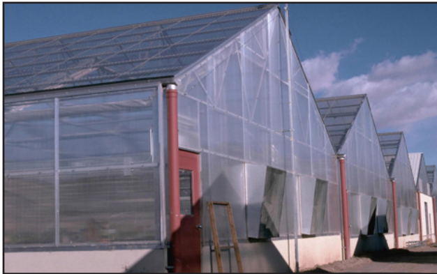
EXTERIOR OF GLASS-COVERED CONVENTIONAL GREENHOUSES.
