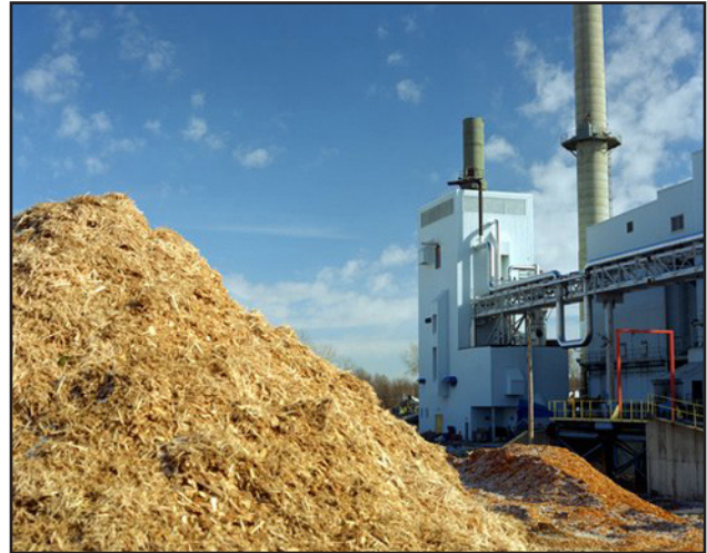
WOODY BIOMASS STOCKPILED FOR USE AT AN ELECTRIC PLANT.
