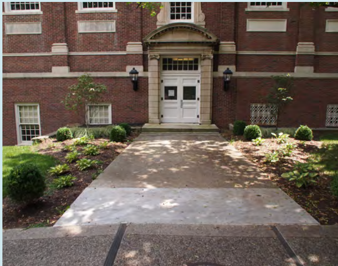
Existing entry to Margaret I. King Library
