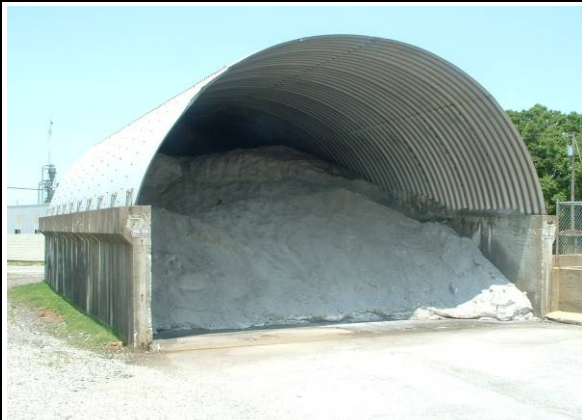
Storing rock salt in a covered dome helps to protect surface and ground water from chloride contamination.
